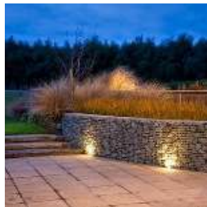
Local materials - gabion walls with river stone
